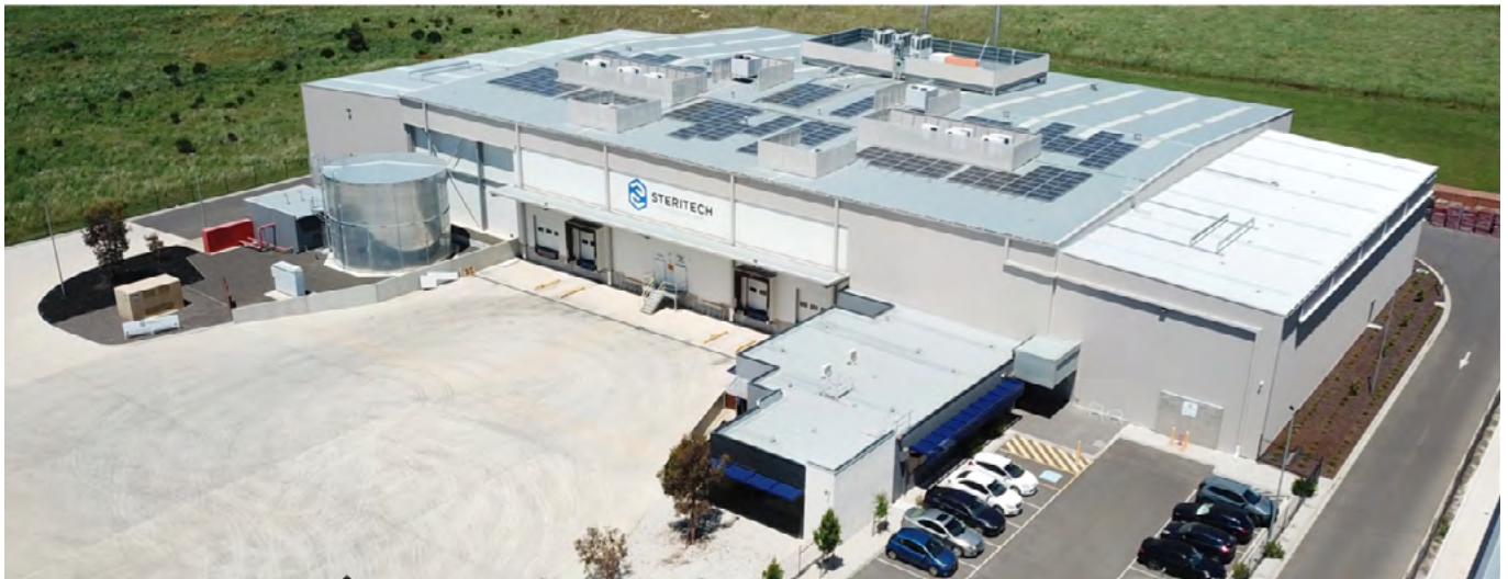
Steritech X-Ray facility in Melbourne. The solar panels pictured generate enough renewable energy to offset all the domestic fresh produce treatments at the facility last year. Steritech is in the process of expanding this solar system to be four times larger, keeping pace with forecasted growth of produce treatments at the site. Photo: Steritech.
