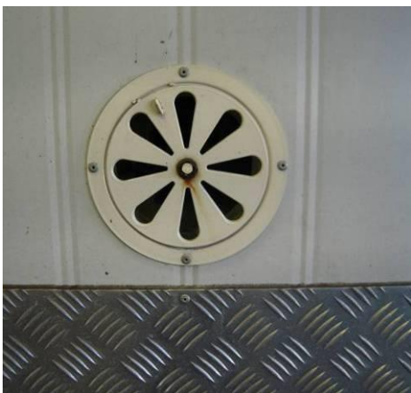
Outlet vent is placed near the floor and can be closed when not flushing the room
