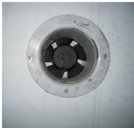
A fan connected to the outlet vent helps to flush the room
