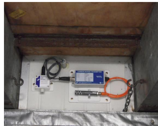
For the controlled monitoring system, a carbon dioxide sensor opens the vent when the level reaches 1%
